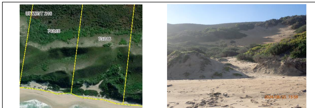
Fig. 14. Two blowouts are evident on the seaward foredune, Portions 73 & 74.
