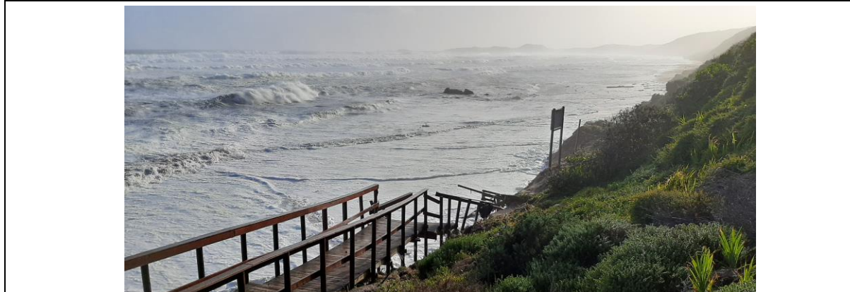
Fig.15. September 2023 storm surge, which washed away the Brenton on Sea beach walkway.
